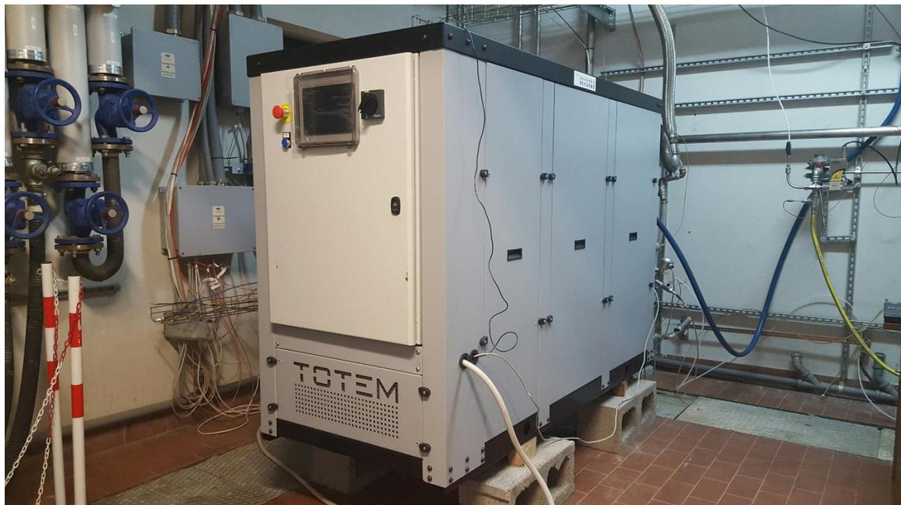
Figure 1. TOTEM 20 under testing in the Laboratory of Micro-Cogeneration at Politecnico di Milano.
